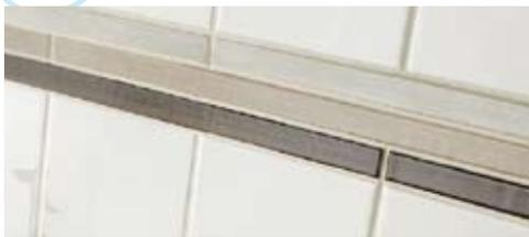
**Porcelain stoneware** Dust-pressed ceramic tiles with water absorption levels less than 0.5% and high mechanical and chemical characteristics. The surface of these tiles may be glazed or unglazed. Often specified for exterior installations, they are also referred to as fully vitrified.
